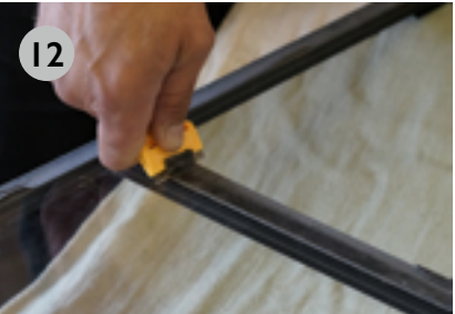
If reusing a glazing unit, residual tape must be cleaned off this too.
