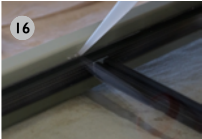
Before reapplying the internal beading apply a strip of silicone to the gap between the glass unit and the sash frame on the bottom rail and 100mm up the sides.
