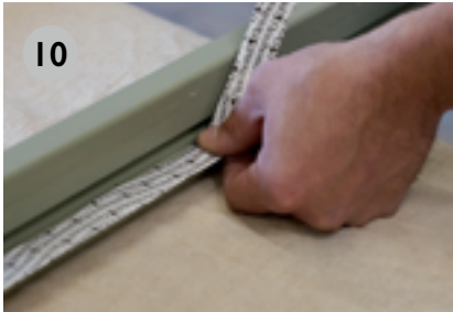
Once all the old glazing tape has been removed, apply Tremco Glazing Tape to the top rail and stiles of the sash.
