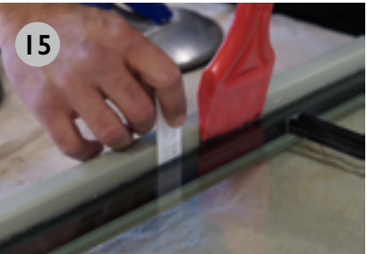
It may be necessary to use a glazing shovel to gently move the glass unit to allow for the placement of the packers.
