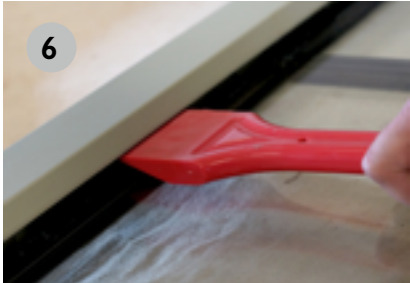
Once all the seals have been cut, prise the glass unit away from the sash frame using a glazing shovel.
