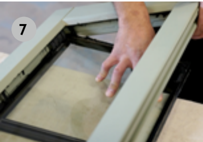
Separate the glass unit from the sash frame and place to one side.
