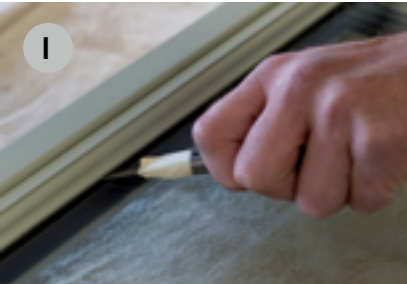
Use either a Fein tool or a craft knife to cut through the seal on the internal bead.
