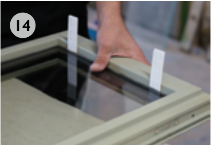
Once happy with the fit, remove the tape backing and fit the glass unit in place. Ensure the glass is fully bedded on the glazing tape.
