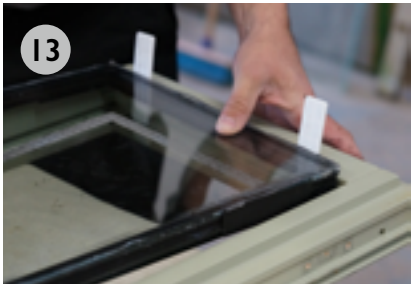
Use the original packers to align the glass unit in place before removing the backing from the new bonding tape.
