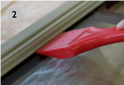
Use a glazing shovel to carefully ease out the glazing bead.
