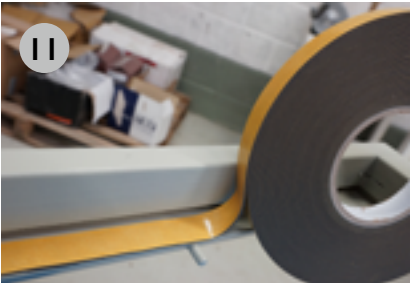
On the bottom rail apply Tremco Glazing Tape leaving a 2-3mm gap between the tape and the edge of the sash.
