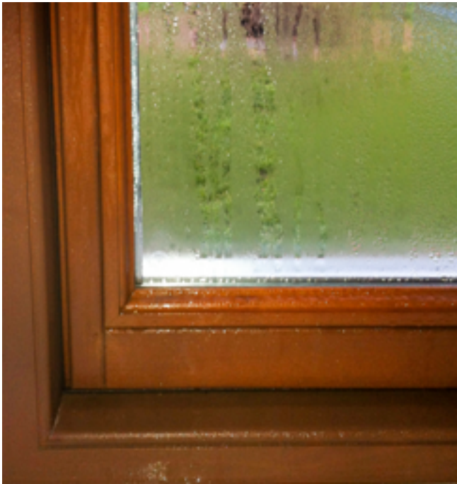
Highlighting damage caused by inadequate ventilation
