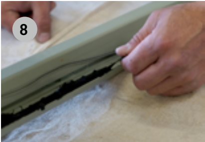
Remove any residual bonding tape and sealant from the sash frame.
