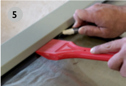
Use either a Fein tool or a craft knife to cut through the external seal. A glazing shovel should be used to increase the gap, to ensure the blade does not damage the paintwork.
