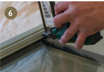
Reapply the internal beading using pins and bar tape to secure the strips in place.
