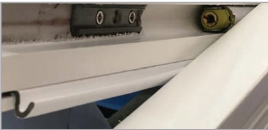
Figure 07: Screw locations for a top sash S2 system
