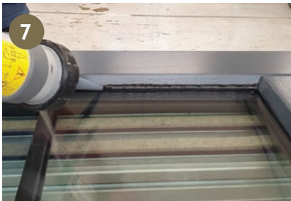
On the external face, apply Otto sealer : on a door, seal all around the perimeter and on a sash across the bottom rail only.
