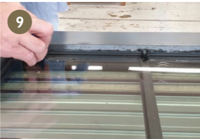
Use a silicone profiling tool to remove excess sealant. If any silicone smears remain, wait until the silicone has cured before removing with a suitable wipe; e.g. Repair Care Easy Q Wipes or Everbuild Multi Use Wonder Wipes .
