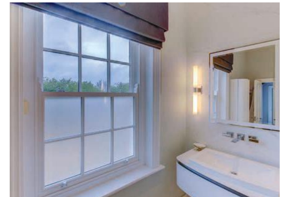
Half obscured glass and bottom sash horns
