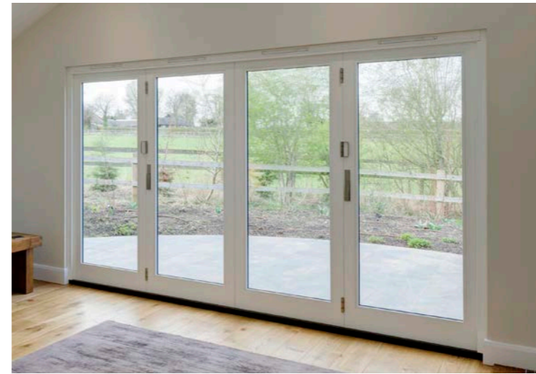
Flush casement windows with classic collection hardware in satin chrome, and discrete trickle vents.
